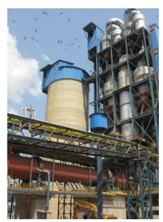
Using these modern heat recycling systems in this way, we can heat the raw material to about 900C before it enters the kiln, thus reducing its time in the kiln itself and the amount of fuel used to convert it into clinker.
